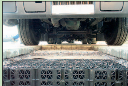
Picture: ENREGIS/Permavoid system. Truck accessible with only 15 cm earth coverage.
