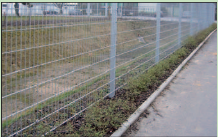
Picture shows high efforts to secure a vegetated swale
