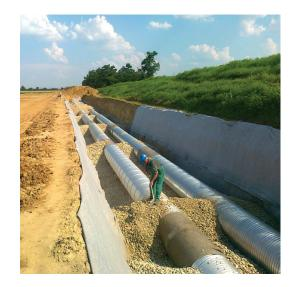
The bed of granular fill is lined with either an impermeable membrane or a geotextile liner, according to local conditions and requirements. Bentonite is particularly suitable with Twinstore, as it seals on wetting. Furthermore, the water is cleaned as it passes through the granular fill. Like any PURECO stormwater attenuation tank, Twinstore can be fabricated to an infinite variety of layouts, unlike concrete chambers or cellular systems which are limited by size and shape.
